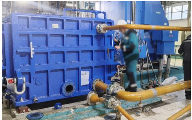
替换后的新齿轮箱 New gearbox after replacement
